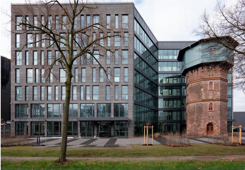
The new company headquarters of ISRA VISION at Frankfurter Str. 112 in Darmstadt
